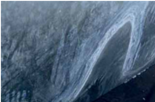
Example: White rust on a bench following incorrect temporary storage on the building site.
